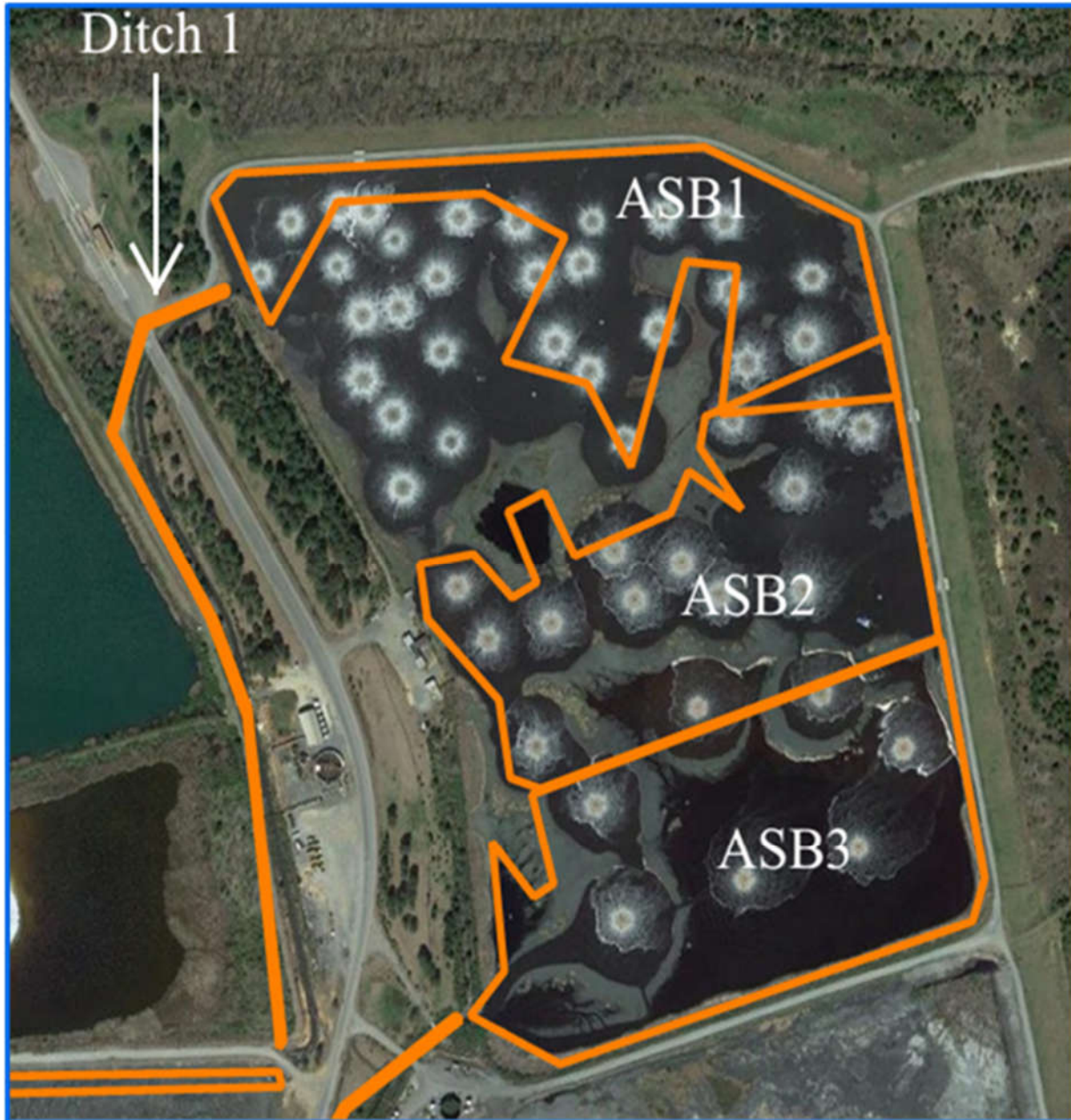
Figure 2. Note the Large (18-acre) dead zone where Ditch 1 empties influent and foul condensate into the ASB.
