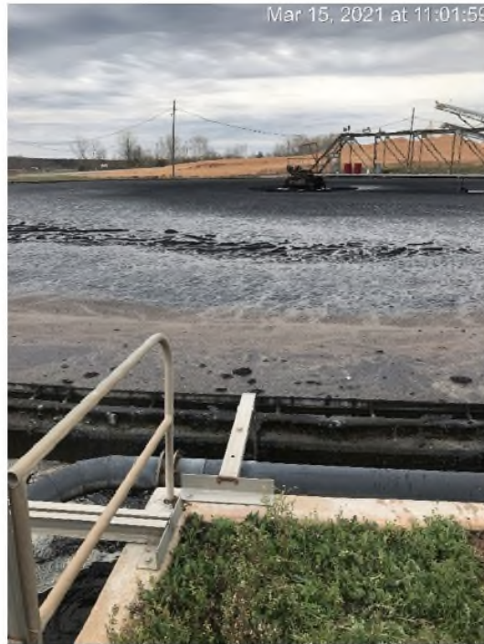
Figure 4. Surface of Primary Clarifier
