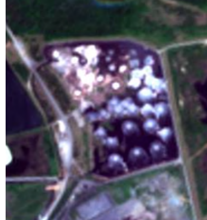
Figure 5b. Severely Damaged ASB Operation in May 2021
